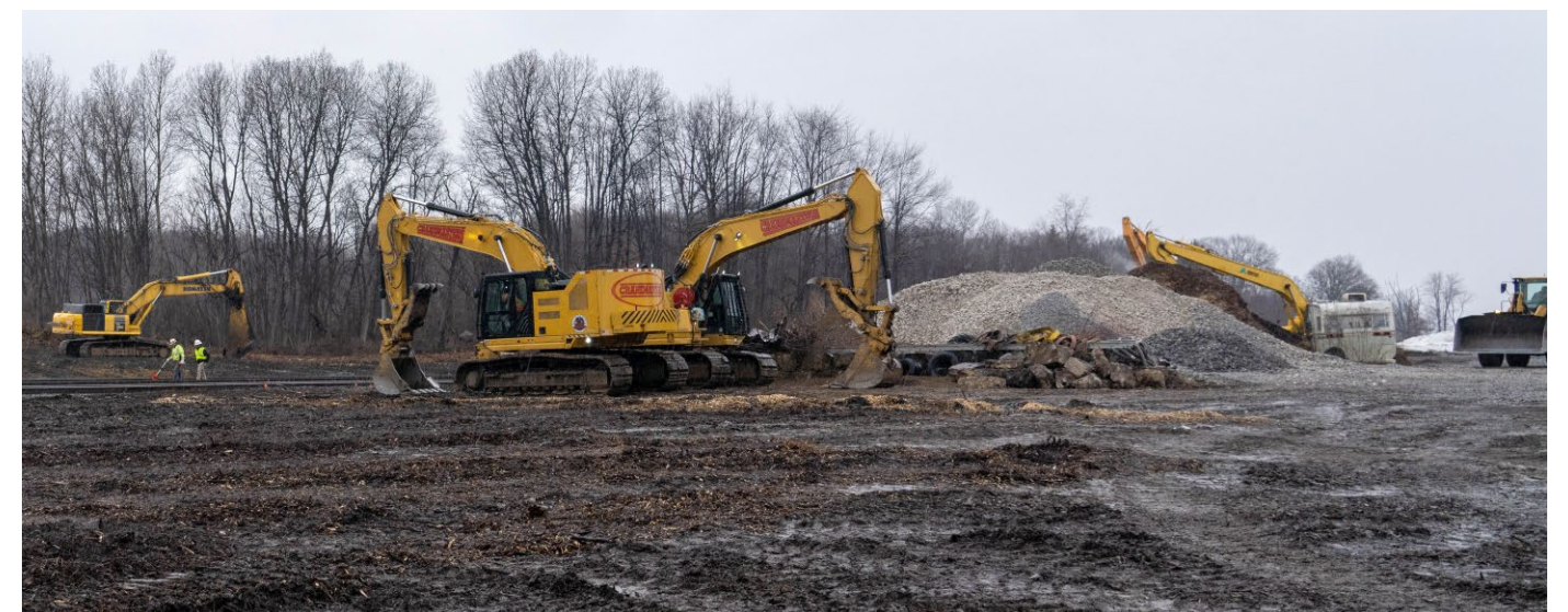
Top Left: The removal of sediment and debris trapped in streams surrounding the Village has led to the return of aquatic life. Norfolk Southern will complete additional treatments to address the sheening that remains. Bottom right: Norfolk Southern completed excavating soil from impacted areas in October.
