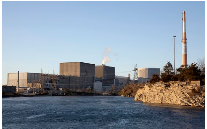
Millstone Power Station.
