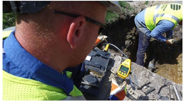
A gas distribution crew performs pipeline testing.
