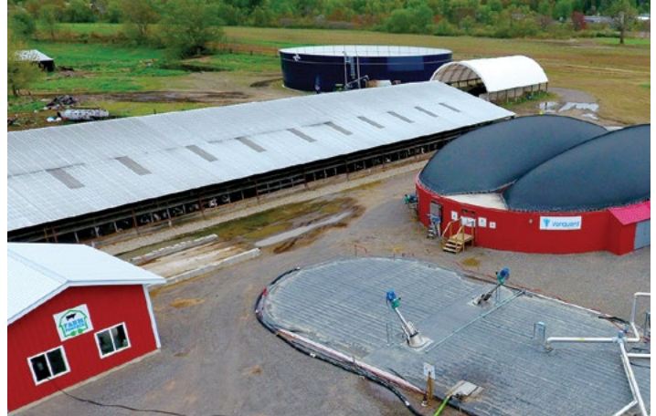
Methane emissions are captured from farming operations for processing into natural gas (photo courtesy of Vanguard).
