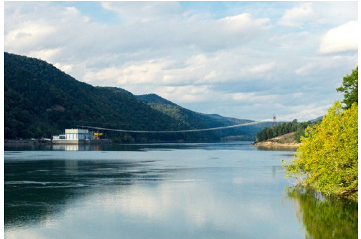
Bath County hydro pumped-storage facility.
