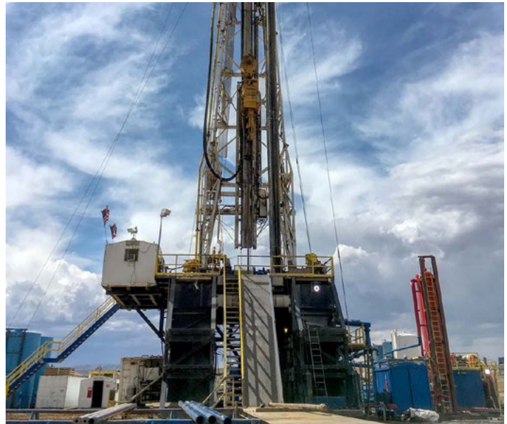
Questar Pipeline also installed flares as a method to achieve additional savings in 2019.
