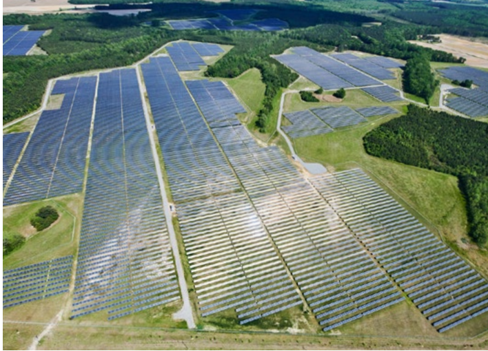
Dominion Energy’s Southampton Solar Farm, consisting of more than 385,000 solar modules on approximately 1,200 acres in Virginia, provides energy to Amazon Web Services.
