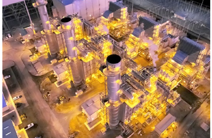
Brunswick County Power Station.
